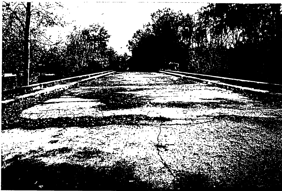
TOP VIEW OF BRIDGE
